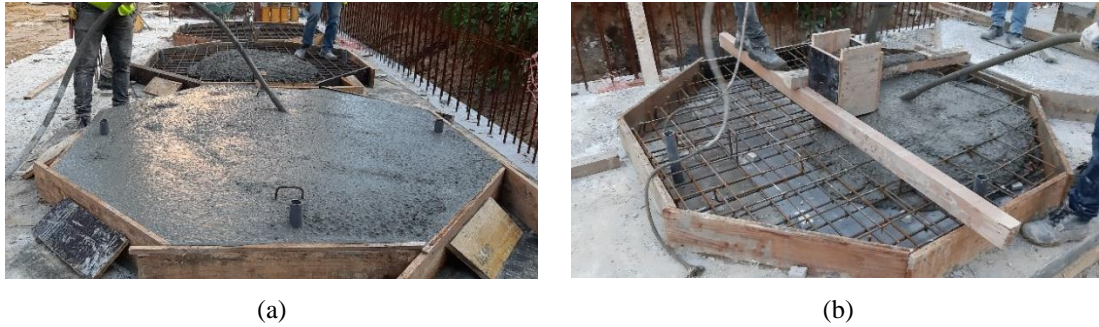
Figure 87. Casting of RC slabs: (a) series PRC, and (b) series PE.
