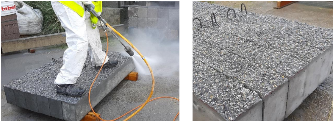
Figure 67. Concrete surface preparation by hydro jetting.
