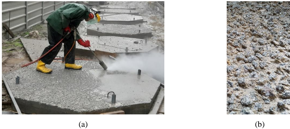
Figure 88. Concrete surface preparation: (a) hydro-jetting process and (b) surface roughness detail.
