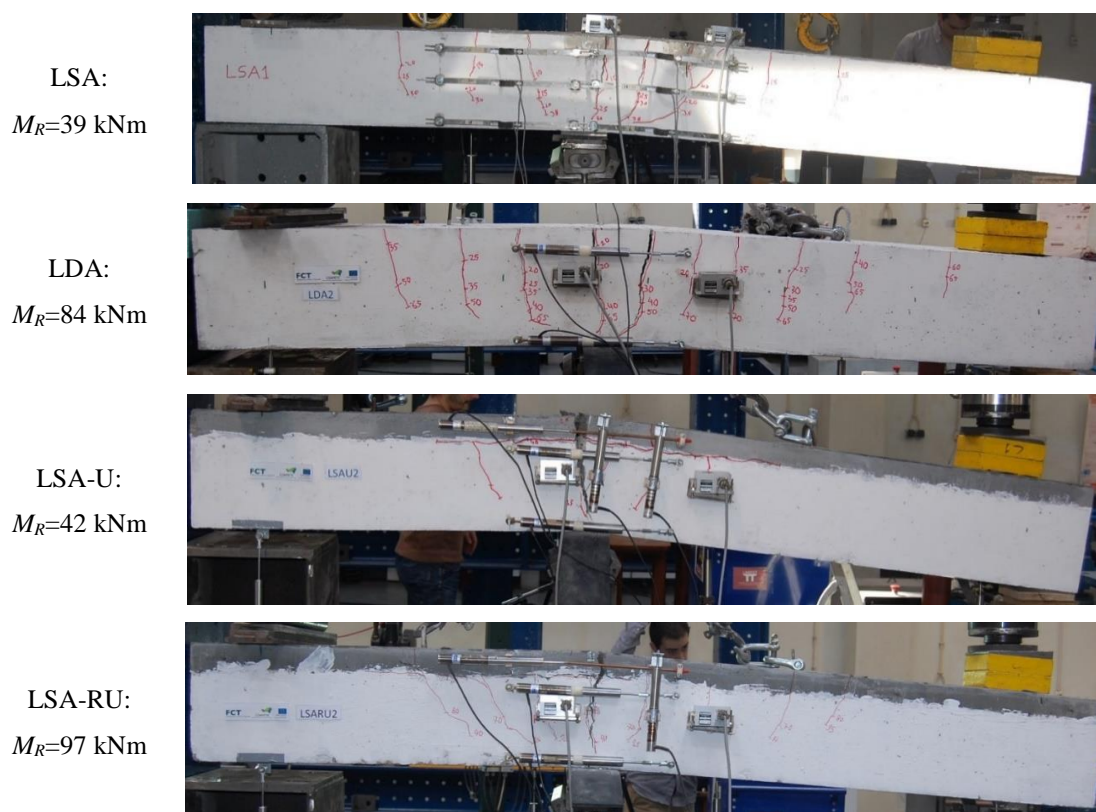
Figure 54. Cracking pattern after the failure of LA slabs.
