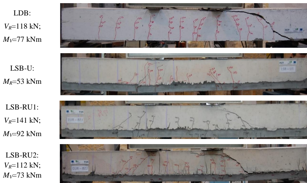
Figure 55. Cracking pattern after the failure of LB slabs.
