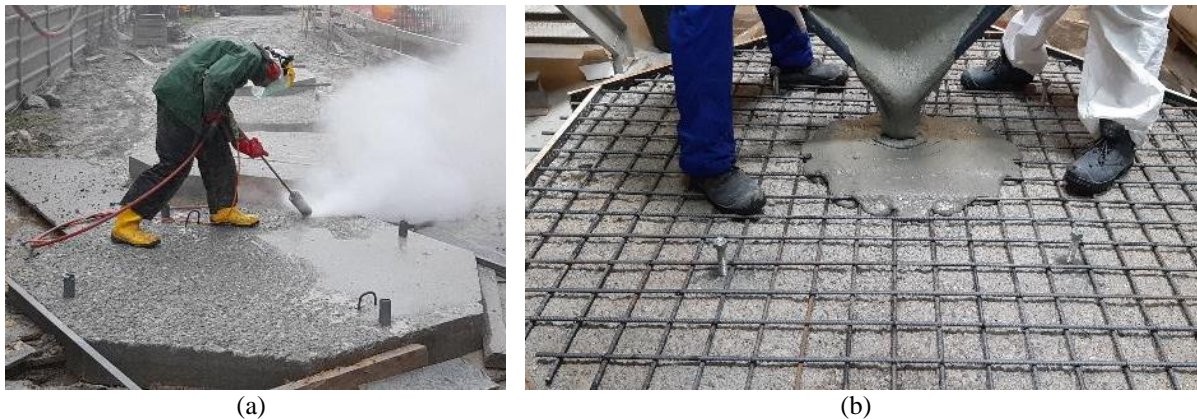
Figure 3. Specimens preparation: (a) hydro-jetting; and (b) UHPFRC overlay casting.
