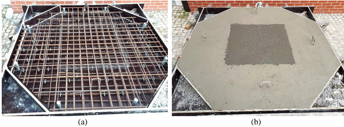
Figure 3 – Casting of specimens: a) formwork and steel net; b) finished product
