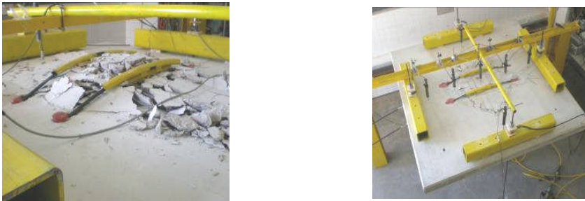
Figure 6: Punching shear failure of the strengthened slab
