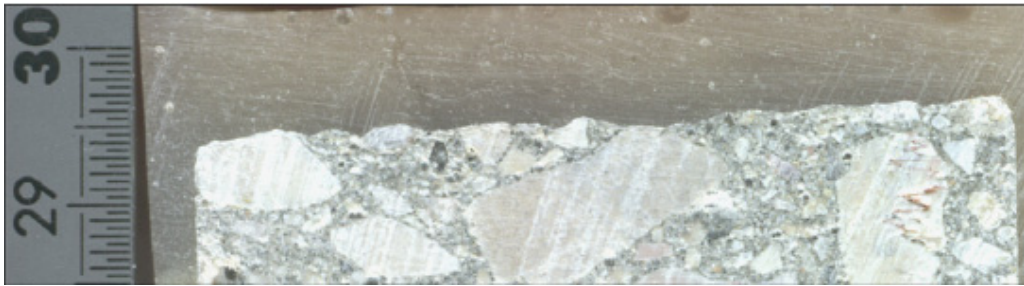
Figure 3.27: Digital image of a concrete specimen (Santos, Julio &amp; Silva, 2007)
