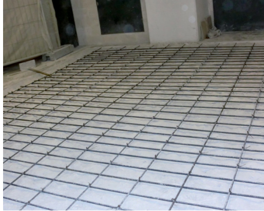
Figure 1.2: Reinforced concrete overlay (Building Visconde de Alvalade )
