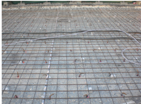
Figure 2.10: Ready to cast overlay (Keesom et al., 2008)
