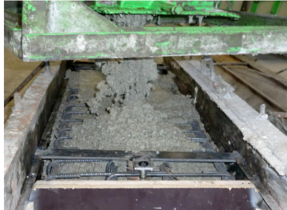
Figure 4.8: Concrete placement
