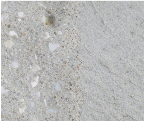
Figure 3.23: Sandblasted surface (left) and left as cast (right)
