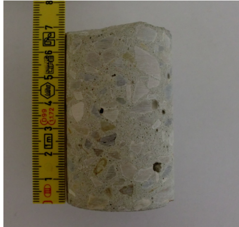
Figure 4.21: Specimen that experienced debonding while drilling the core
