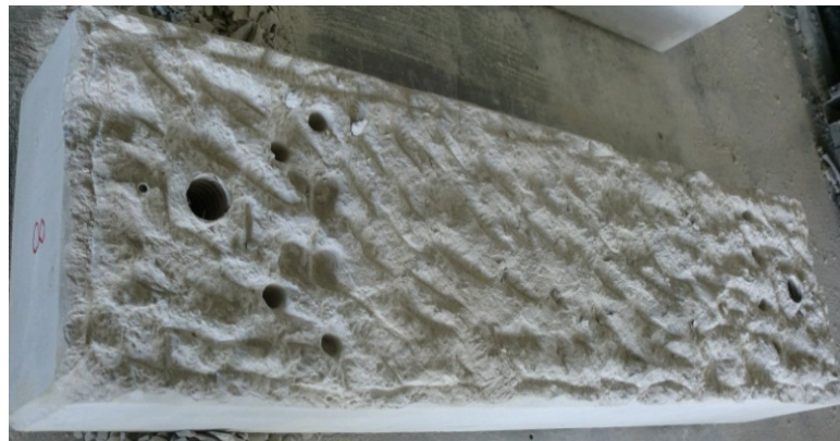
Figure 4.17: Anchorage holes in specimen III.C
