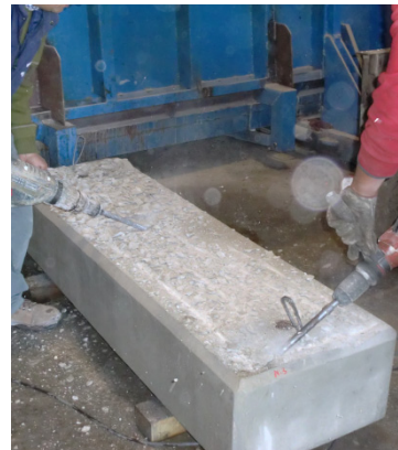
Figure 4.10: Roughening the substrate
