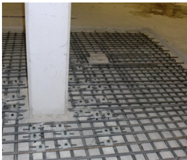
Figure 2.7: Longitudinal and punching shear reinforcement
