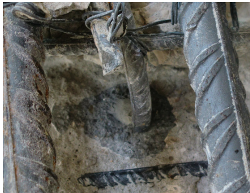
Figure 5.12: Appearance of a grouted dowel, after the beams were tested
