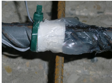
Figure 4.31: Impermeabilized strain gauges
