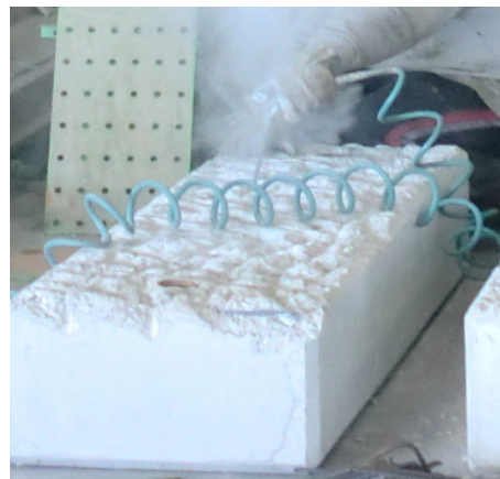
Figure 4.12: Cleaning the holes with compressed air
