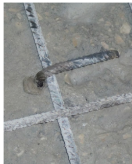
Figure 2.8: Shear connectors crossing the interface
