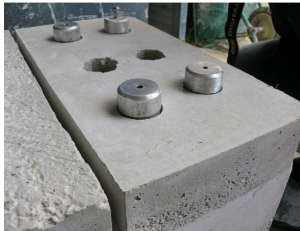
Figure 4.19: Test discs attached with an epoxy adhesive ( araldit® ) to the concrete
