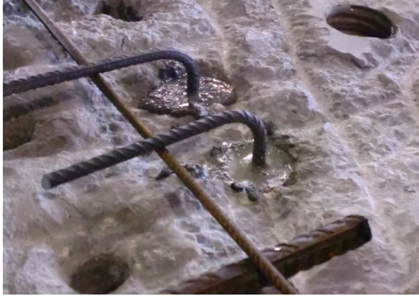
Figure 4.13: Post-installed reinforcement (SM II)
