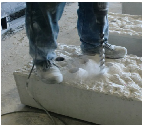
Figure 4.11: Perforations for the post-installed reinforcement
