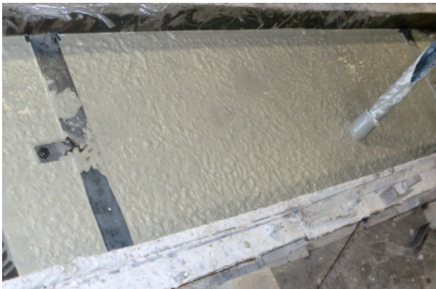
Figure 4.9: Concrete vibration
