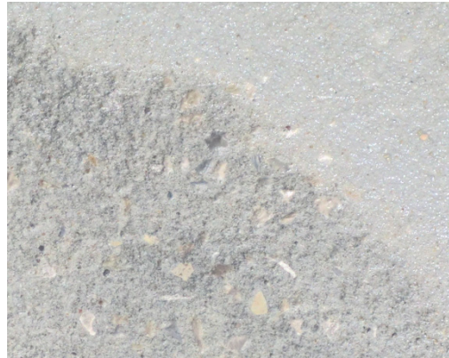
Figure 3.24: Wirebrushed surface (left) and left as cast (right)
