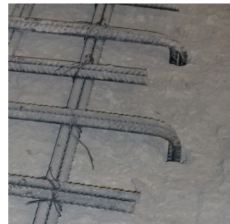
Figure 2.9: Anchorage of the longitudinal reinforcement
