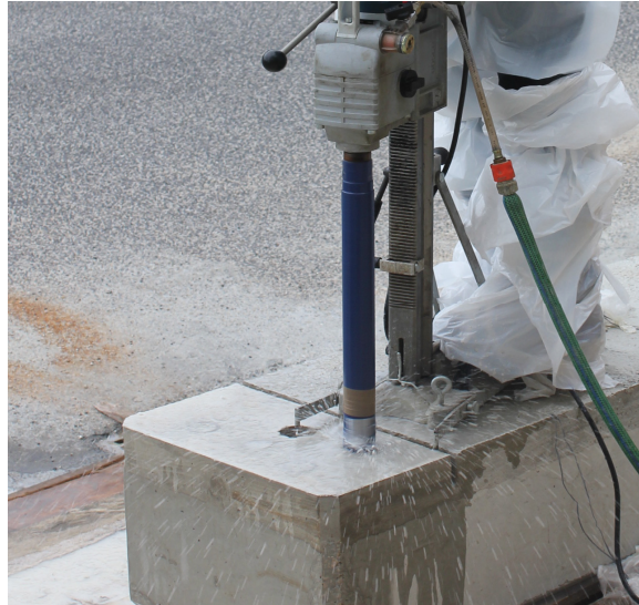
Figure 4.18: Drilling the cores
